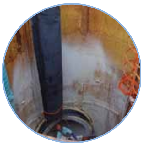
Inserting a folded pillow plug
