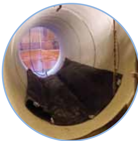
Placing – pillow plug should be positioned horizontally
